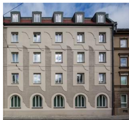
Munich. Housing block renovation.
