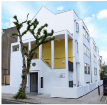
Artic Street, Housing Coop, Camden
