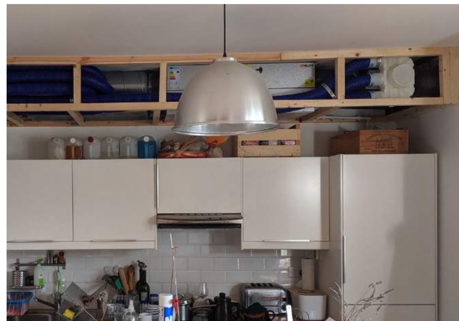
Installation of a whole house mechanical ventilation system with heat recovery in a flat as part of a retrofit. In this case installed in the ceiling above a kitchen.
